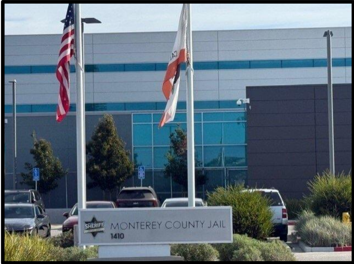
Monterey County Jail Administrative Entrance
