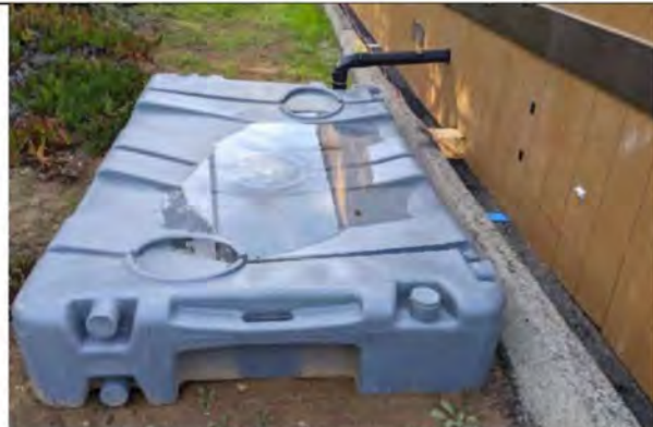
Septic system for modular trailer
