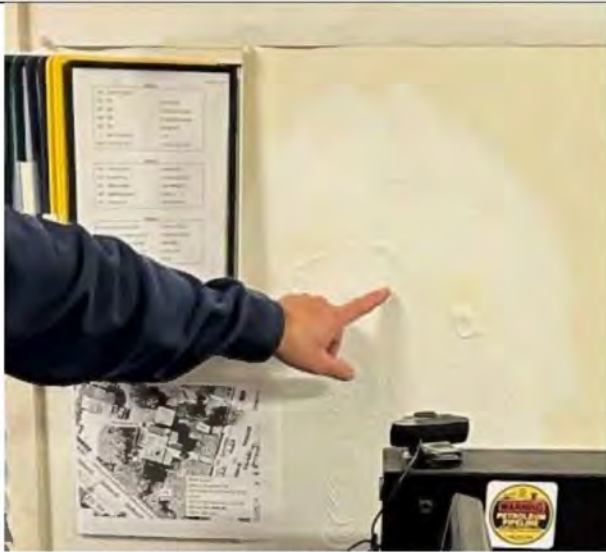
Bubbling paint after two weeks
