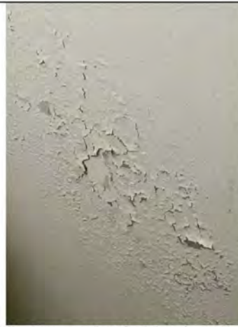
Kitchen paint flaking/peeling
