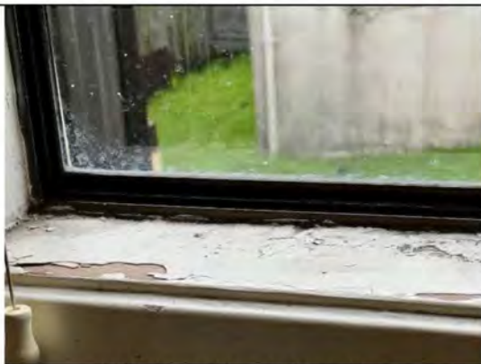
Window sill paint peeling
