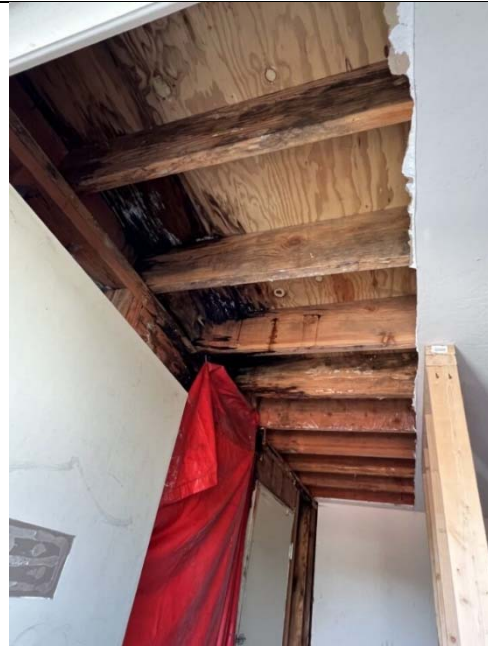
View inside abandoned training tower
