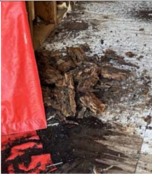
View inside abandoned training tower
