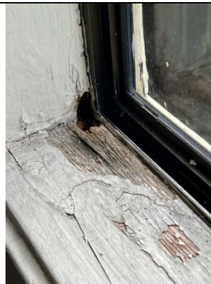
Kitchen area windowsill
