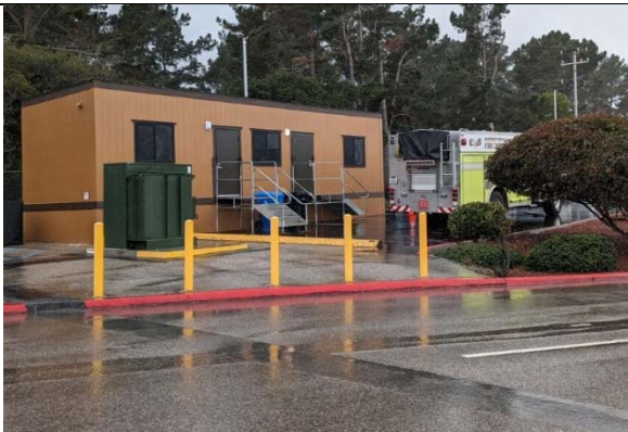
Modular trailer "fire station" at airport
