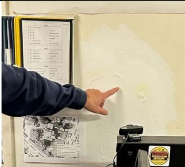
Bubbling paint after two weeks
