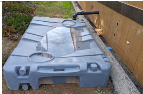
Septic system for modular trailer
