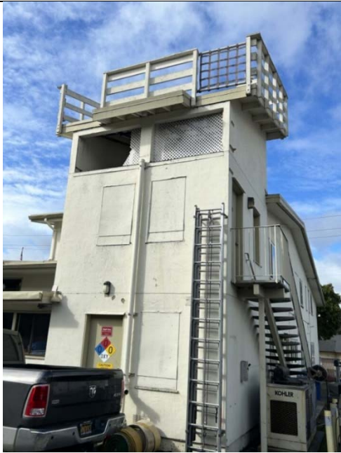
Abandoned training tower
