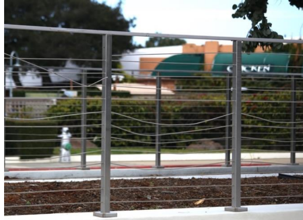
NFBPIP Railing: February 18, 2021
